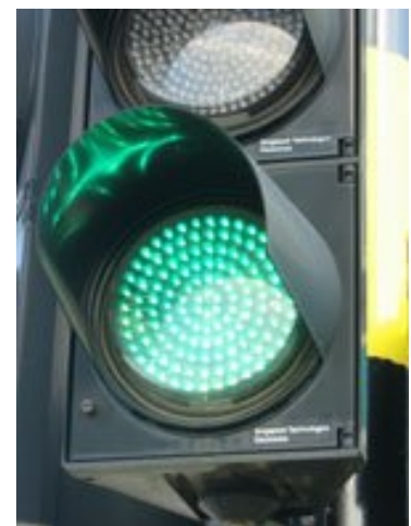
Retrofitted LED Stoplight
